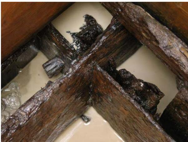
Figure 129. Corner of the wooden well lining showing horizontal planks connected by a simple lap joint, and a wooden peg driven into the corner post through one of the horizontal planks.
