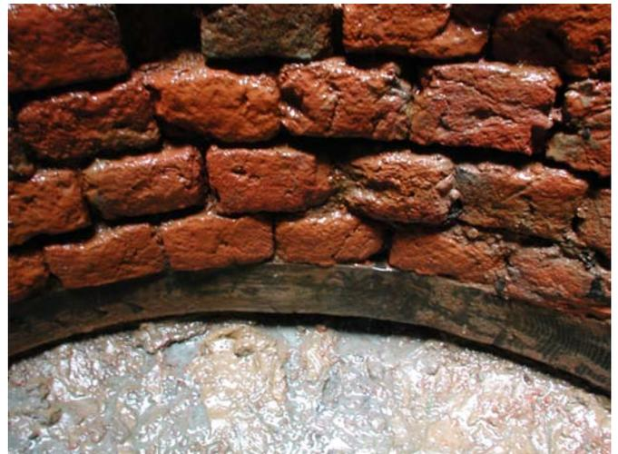
Figure 137. Wooden curb (JR973L) beneath the final course of bricks.
